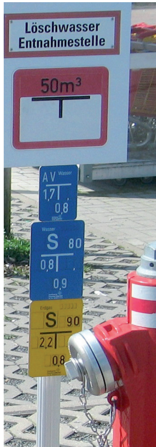
Figure 13: Indication of cisterns with water for extinguishing fires, gate valves (S) for a water pipeline, 80 mm (blue), and a gas pipeline, 90 mm (yellow): The numbers indicate the distance in metres in two directions. kanaldeckel.htm
