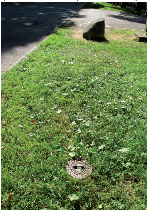
Figure 11: This iron cap indicates the position of a gate valve. In which direction does the water flow through the pipeline? kanaldeckel.htm
