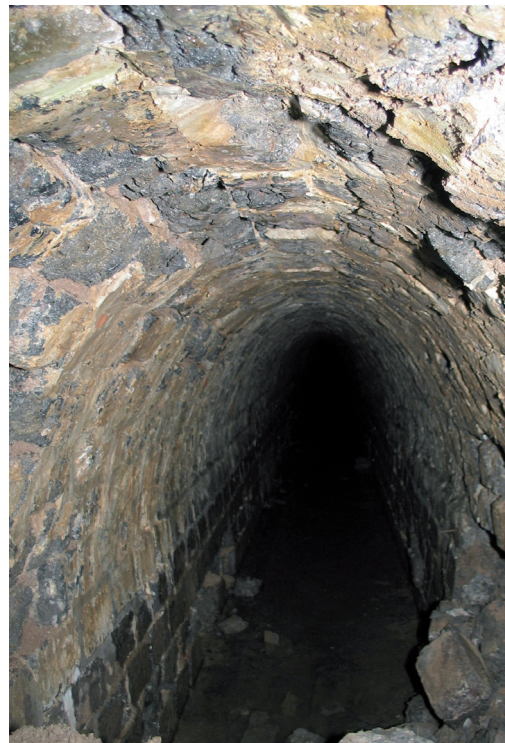
Figure 60: This drainage gallery from the mining era extends horizontally. marie.htm
