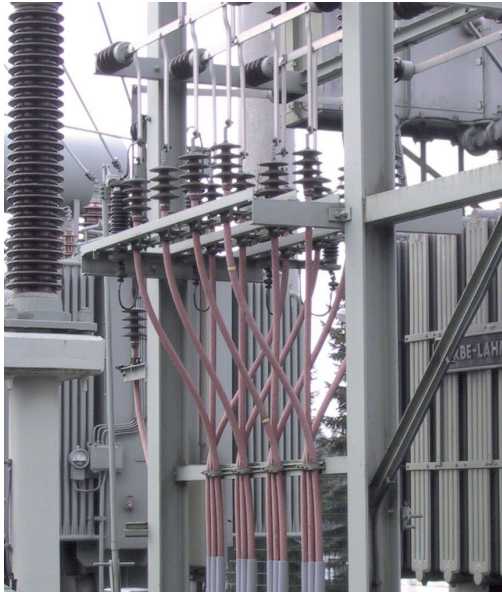
Figure 14: From this substation at the edge of Zellerfeld, electric power is supplied at 20 kV by buried cable. Each of the four individual cables is a bundle consisting of three red cables. stromkabel.htm
