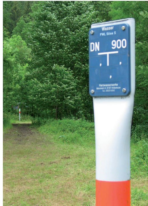
Figure 12: The direction of flow in this long-distance water pipeline with a diameter of 900 mm is clearly marked for easy visibility. The next post is located on the left within the range of sight in the background. This is a good opportunity for investigating the perceptible properties of a pipeline and for training purposes.
