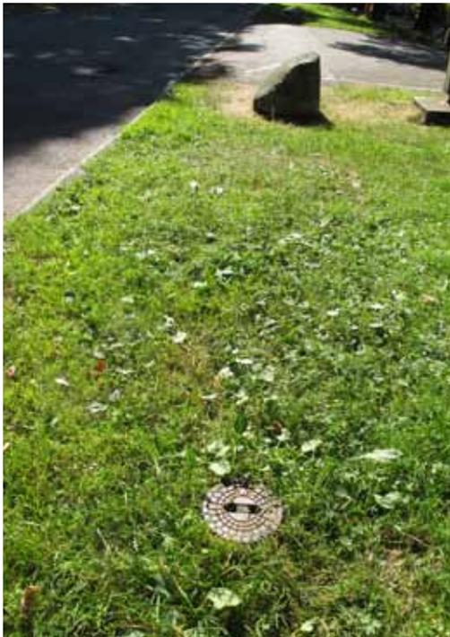
Figure 11: This iron cap indicates the position of a gate valve. In which direction does the water flow through the pipeline? [kanaldeckel.htm](http://kanaldeckel.htm)
