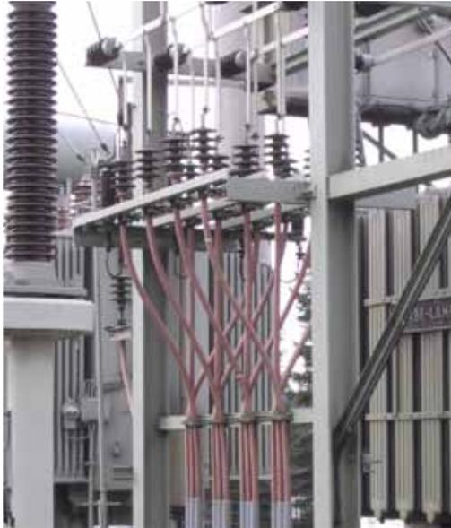
Figure 14: From this substation at the edge of Zellerfeld, electric power is supplied at 20 kV by buried cable. Each of the four individual cables is a bundle consisting of three red cables. [stromkabel.htm](http://stromkabel.htm)
