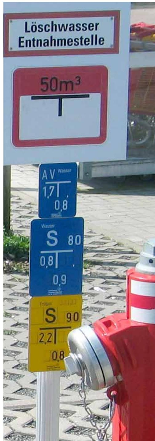
Figure 13: Indication of cisterns with water for extinguishing fires, gate valves (S) for a water pipeline, 80 mm (blue), and a gas pipeline, 90 mm (yellow): The numbers indicate the distance in metres in two directions. [kanaldeckel.htm](http://kanaldeckel.htm)
