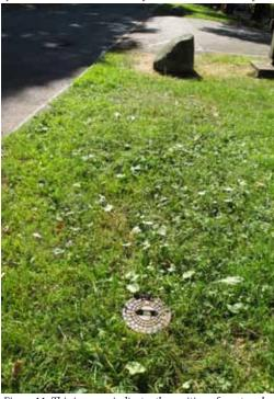
Figure 11: This iron cap indicates the position of a gate valve. In which direction does the water flow through the pipeline? kanaldeckel.htm
