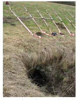
Figure 61: The drainage gallery emerges on a slope. The altitude of the terrain over this cavity increases slightly.
